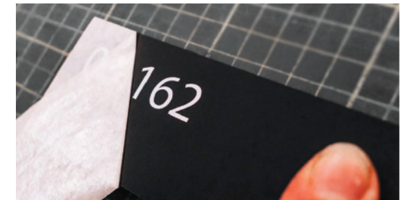
Vinyl numbering being applied to header
