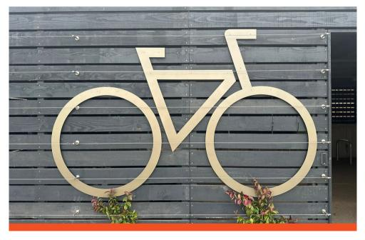
Crafted using 3mm aluminium, fret cut with a painted finish. This is a smart look for an employee storage solution, providing a safe space for bicycles at the workplace and encouraging a viable commuting method to help reduce traffic congestion and carbon footprint.
