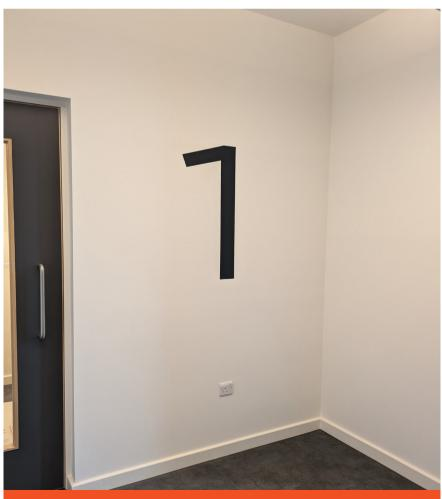
The internal floor numbering is bold and striking. Acrylic fret-cut floor numbers are fixed to ultra-modern sustainable wooden batons using hidden fixings. Vinyl painted floor numbers cut using a computerised stencil template are adhered directly to the wall.
